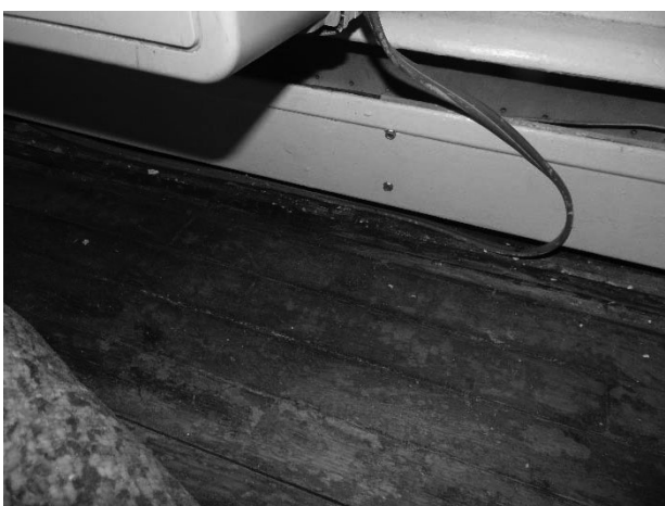
Water damage and mold growth under the bedroom in-wall Hvac system on hardwood flooring and wall materials
