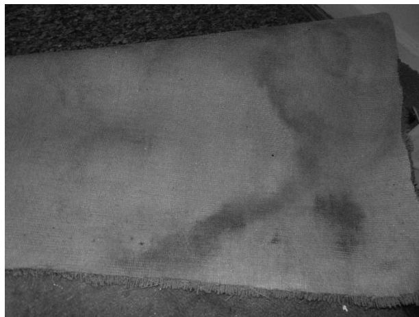
Visible mold growth and water staining to the bottom surface of the bedroom carpeting
