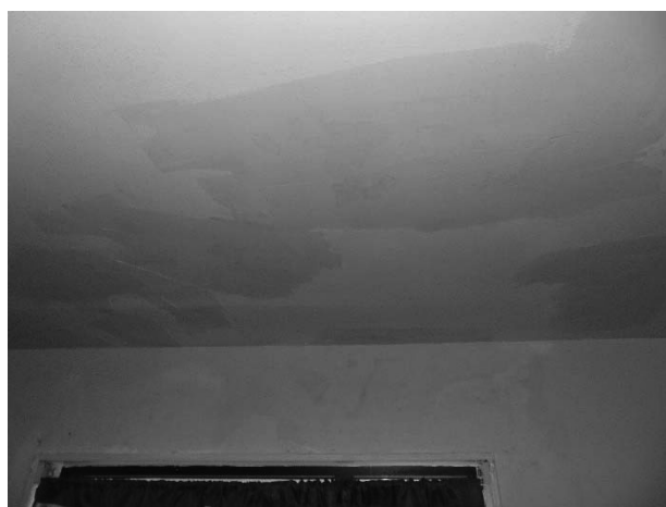
Water damaged materials painted over in the bedroom
