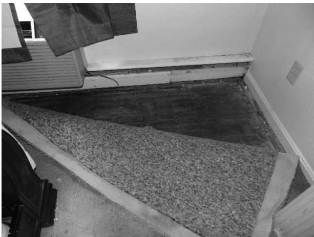
Visible mold growth and water damaged flooring materials
