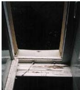
Leaky window - mold is beginning to rot the wooden frame and windowsill.
