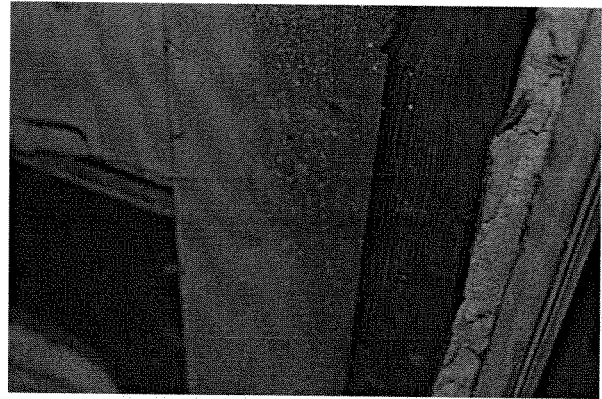
Mold growth painted over on framing
